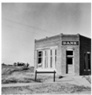
Failed bank, Kansas, 1936
